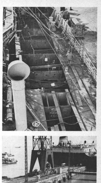
NORTH YARD: Renewing main deck plating and cargo tank internals. 400 tons in 41 days 4 drydocks up to 18,000 t.d.w.
