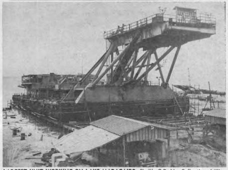
**LARGEST UNIT WORKING ON LAKE MARACAIBO,** Shell's G.P. No. 9 floating drilling barge and work-over rig, is hauled out at the Varadero Y Astillero del Zulia Compania Anonima, Maracaibo, Venezuela, shipyard for repairs. The unit was enlarged and the cantilever platform added in 1966 by the same shipyard. With the derrick and rotary removed, the barge, as shown, weighs 2,619 tons.
