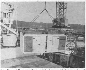
Loading of Dorsey refrigerated stores container equipped with Thermo-King units is tested at the shipyard. Stores containers are pre-loaded on the pier, thus reducing turn-around time of ship.
