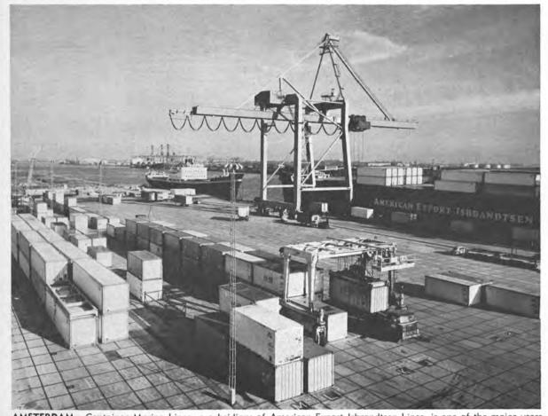
**AMSTERDAM**—Container Marine Lines, a subsidiary of American Export Isbrandtsen Lines, is one of the major users of Container Terminal "Amsterdam", a 164,000-square-foot facility able to accommodate 1,500 twenty-foot containers at one time. The crane shown has a 50-ton lifting capacity and an outreach of 118 feet over the water and 144 feet over the quay. This terminal also is the trans-shipment center for containers coming by rail to Amsterdam.
