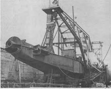
A unique "teeter-totter" method, devised by the rigging department foreman at Bethlehem Steel Corporation's San Francisco shipyard, was employed to unstep the 105-footlong digging ladder on the hydraulic suction dredge Franciscan. The dredge is shown on drydock at the yard before the ladder was unhinged and sponsons welded to the hull.
