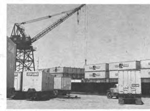
Containers being handled by one of three 60-ton gantry cranes at Philadelphia terminal. Since 1968 containers have been stuffed at this facility.
