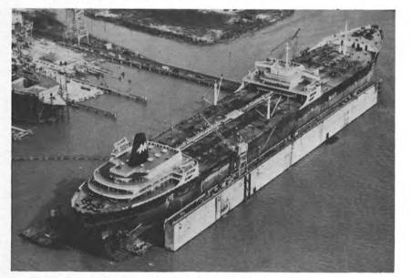
38,000 ton floating dry dock; Chester, Pa. Crandall-Type hull design reduced dead weight 800 tons
