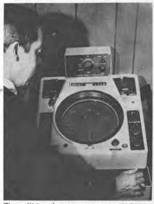
The collision threat assessment unit is provided as an attachment for the standard marine radar, true or relative motion.
