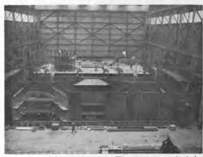
Vertical module construction. This unique method facilitates positioning of subassemblies and permits concentration of labor and tools in a small area.
