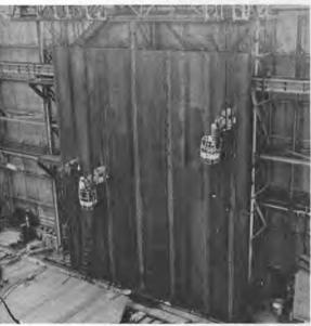
Joining panels by use of the electro-gas welding process.
