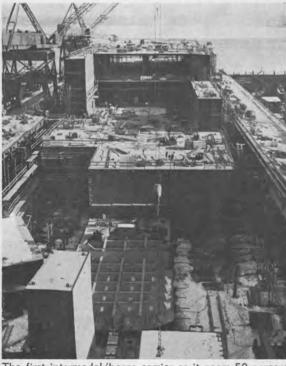
The first intermodal/barge carrier as it nears 50 percent completion of its steel structure in only six months after keel laying at the Quincy yard.
