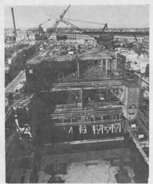
This stern view shows the cantilever sections extending beyond the stern. In the foreground are the first two girders for the elevator platform.
