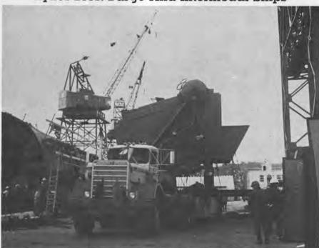
The first of two B&W boilers for the Doctor Lykes is moved into position for lifting aboard the vessel at the Quincy Division shippard of General Dynamics in Quincy, Mass.
