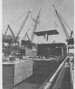
Landing a 95-ton upper deck section on the Doctor Lykes on January 20 brought the steel erection to over 50 percent completion for the first ship.
