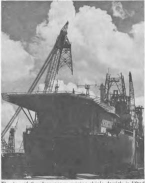
The top of the deep-ocean mining ship's derrick is lifted into position by Sun Ship's floating derrick barge.
