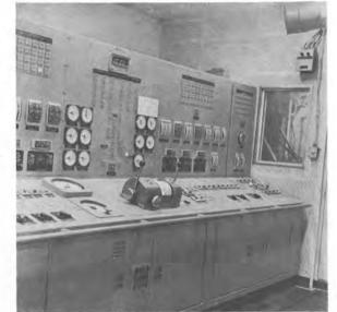
Main engine console is located in a sound-proof room. View was taken looking forward and toward starboard.
