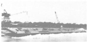
Side launching of 330-foot hull for a floating grain transfer facility took place recently at Bergeron Industries' yard in Braithwaite, La.
