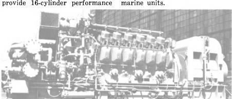
12-cylinder generator set built by Alco produces 2,000 kw at 1,200 rpm.
