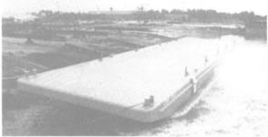
A significant event occurred recently at Bergeron Marine when the barge CMS-563 (shown above) slid down the launchways at the company's Port Bienville facility. The 120-foot by 30-foot by 7-foot steel deck barge built for Central Marine Service, Inc., New Orleans, was the 100th vessel constructed at the Mississippi yard.
