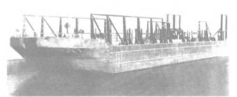
Type: • Ocean unmanned service • Grade "B" bulk cargo • Dunnaged deck for general cargo USCG: · Documented with "Certificate of Registry" · Operating "oceans" · Official No. · 280390 · Net: 2045-6ross: 2045 · Length: 260 · 0 Breadth · 52 · 1 · Depth: 18.3
