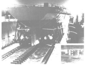
Ship at Pori rests on Hydranautics roller beams prior to movement onto floating dock. Insert shows positioning jacks that are used to align ship sections in preparation for ship assembly welding. sitioning jacks for vertical lift and horizontal move during positioning of ship sections; and accompanying interconnecting hoses with quick disconnects.
