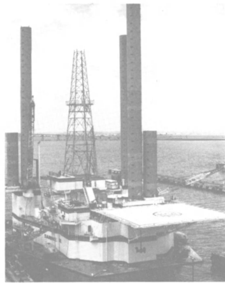
Jackup drilling rig Sabine III, owned by Houston Offshore International, was commissioned recently at Bethlehem's Sparrows Point yard. When completed, rig will be towed to Gulf of Mexico where it will drill for Exxon Company, U.S.A.
