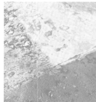
Heavily rusted deck (below), after water blasting (left), and "white-metal" clean after water-sand blasting (right)."
