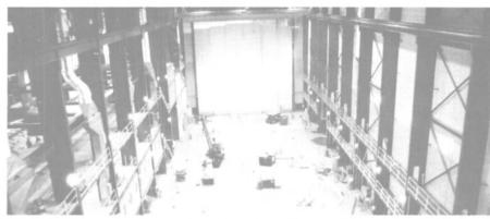
Gangways from the mezzanine on the left and from walkways on the right with provide quick access to ships under construction and eliminate the need for traditional scaffolding. At the front and rear of each bay, 70-foot high doors, consisting of 6 sliding panels, open to a width of 65 feet.
