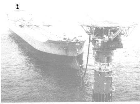
Rising 643 feet above seabed, unmanned articulated tanker loading platform loads produced crude into shuttle tankers modified to accept bow hose connection. The Statfjord "C" ALP was engineered, constructed and installed by Single Buoy Moorings, Inc., of Switzerland.
