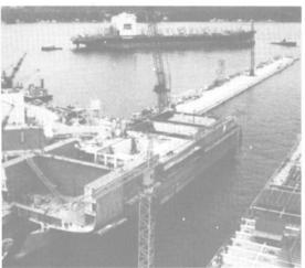
Bay Ship Hull No. 736 (foreground) being floated forward in graving dock. In background is Hull No. 735, having just been floated out of the dock, being towed to an outfitting pier for completion.
