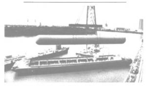
ONE OF TWO LPG (liquid petroleum gas) tanks built at the Beaumont yard of Bethlehem Steel Corporation is being loaded onto a barge for inland waterway service. Built for Fredeman Shipyard, Sulphur, La., each tank measures 176 feet long, almost 17 feet in diameter, and has a capacity of 281,000 gallons. Fabrication of the two tanks required a total of 480 tons of steel.
