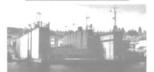
**DRYDOCKED DRYDOCK**—A routine maintenance job on its 500-ton capacity drydock created this not-so-routine right at Marco Seattle when the shipyard lifted the smaller dock in its 1,800-ton counterpart to do the work. Both of the steel drydocks were designed and built by Marco.
