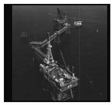
McDermotfs DB50, rear center, sets Production Platform No. 1 deck for Freeport-McMoRan Resource Partners (Limited Partnership) Main Pass Block 200 Sulfur Project in the Gulf of Mexico, completing the western one-third of the 15-platform offshore sulfur mining complex.
