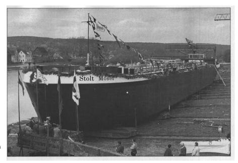
The M/T Stolt Mosel, built by Bayerische Schiffbau GmbH shipyard in Erlenbach, Germany, is one of five 2,100-dwt inland chemical I tankers designed by Stolt-Nielsen to transport bulk liquid along the Rhine.
