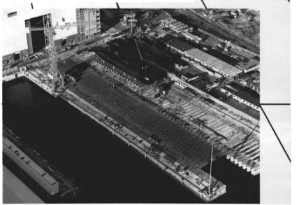
Vickers Shipbuilding and Engineering Works Ltd. Barrow-in-Furness, United Kingdom. Maximum Shiplifting Capacity - 25,000 Tons. Latitude 54.07N Longitude 3.14W.
