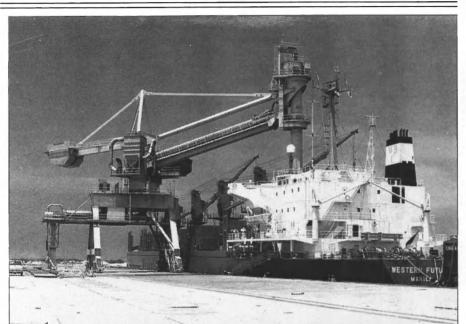
Continuous ship unloader by PWH Anlagen, a company of Krupp Fordertechnik.
