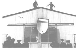
Drop test from the roof of the boatbuilding shed using a plastic rowing boat in 1957.
