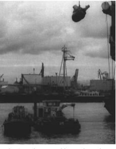
Hydrex's underwater ship repairers dug a trench using a six in. salvage pump. Five days after intense dredging and removal of debris and rocks — a crater of 5 m deep was created under one of the four main propulsion thrusters.
