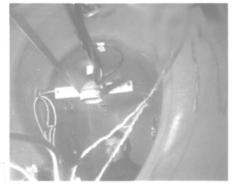
Diver seal technician — bonding lip seal located above, while below the lighting system is the bonding jig.
