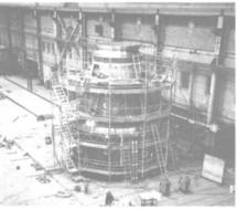
ABS surveyors, onsite at Junoverken AB yard in Uddevalla, Sweden, monitor and inspect the fabrication of industry's first offshore LNG deepwater port buoy
