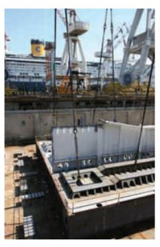
Ponente shipyards in Genoa. This first block, an aft section, measures 55.7 ft. (17 m) long and 72 ft. (22 m) wide, and weighs approximately 500 tons.
